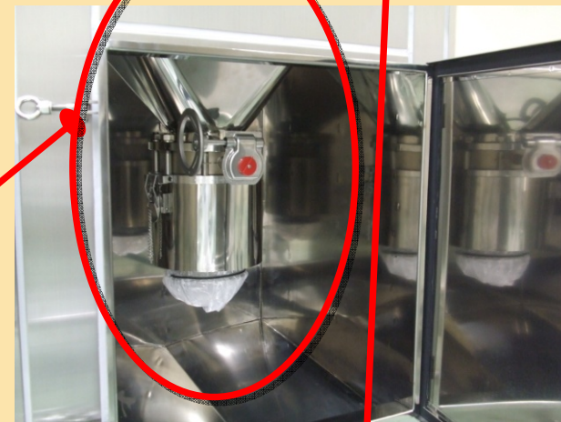
Embedded dust collector in the wall of processing room
